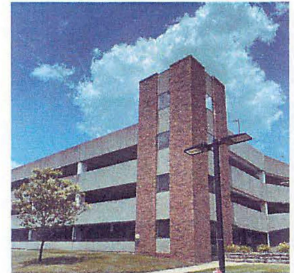
Current Parking Deck at 5th and Lincoln planned for demolition in the next couple of years
