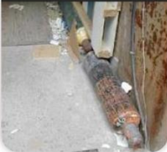
COMPRESSED GAS UNSAFE STORAGE
