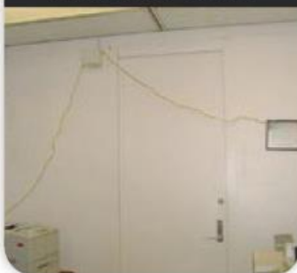
EXTENSION CORDS, NOT PERMANENT WIRING
