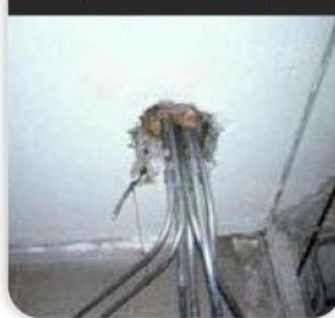
NO FIRE STOPPING IN OPEN PENETRATION
