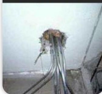
NO FIRE STOPPING IN OPEN PENETRATION
